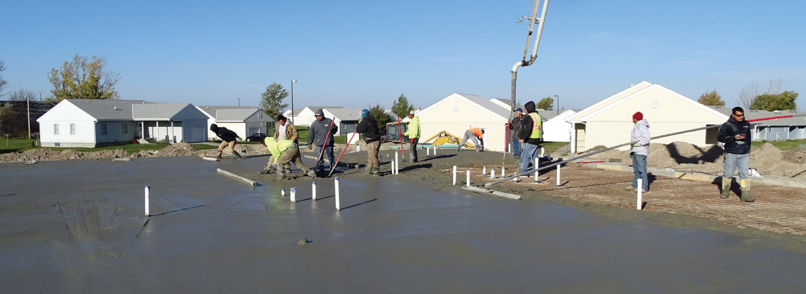
Concrete floor pour at IHS apartment project.
